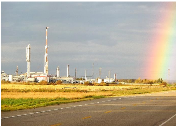
Dunvegan Gas Plant Operated by Canadian Natural Resources Ltd
