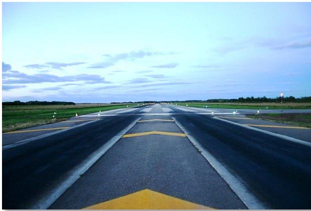
Fairview Airport Runway
